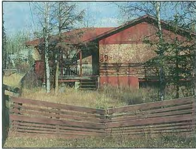
Photo 44: Inadequately maintained zone 1
