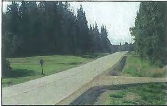
Photo 5: Ditch grass & vacant lot in excellent condition.
